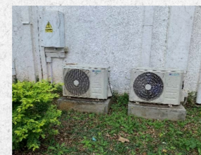
Poor maintenance of AC units
