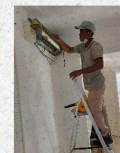
Preventive maintenance in action
