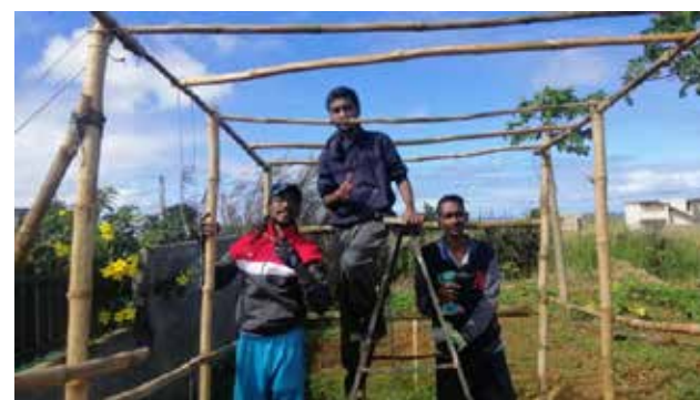
Figure 8: Construction of bamboo greenhouse-recycled materials and bamboo used
